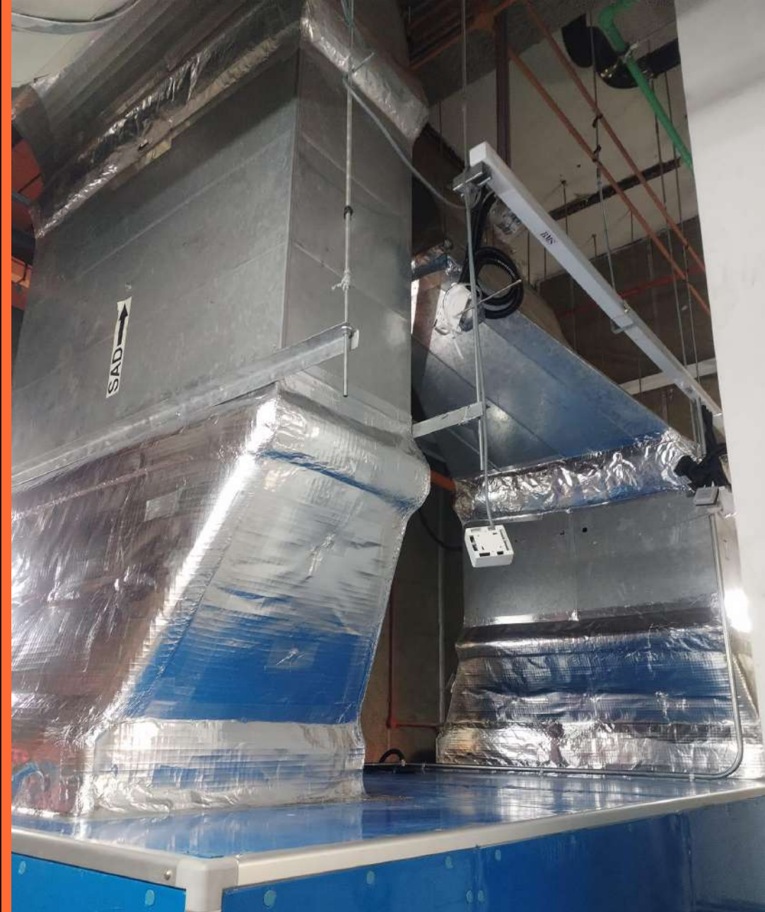
Air handling unit installation
